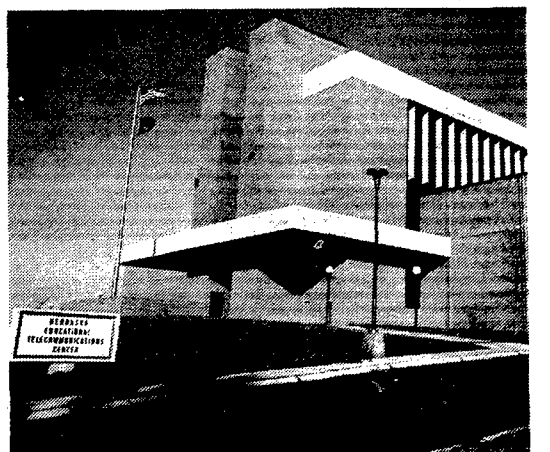
The 2.4 million Nebraska Educational Telecommunications Center at Lincoln, which will be dedicated Sunday, June 4.
